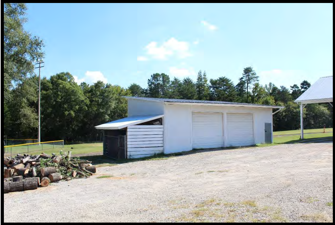
Figure 22: Shed, Mallard Creek School, Looking Southeast.
