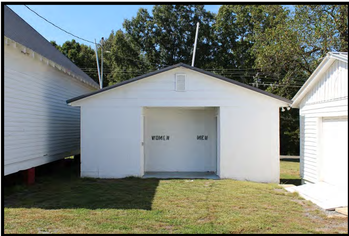
Figure 9: Restrooms, Mallard Creek School, Looking West.
