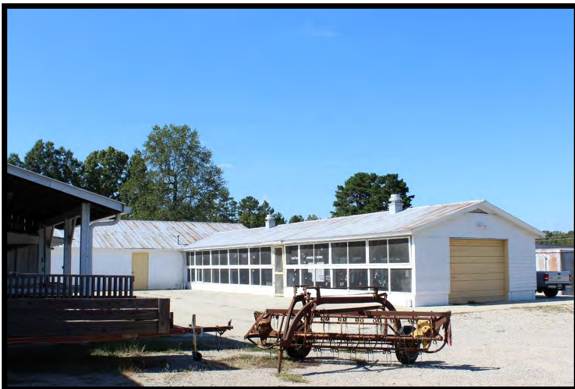
Figure 14: Sandwich Stand and Barbecue Building, Mallard Creek School, Looking Northeast.
