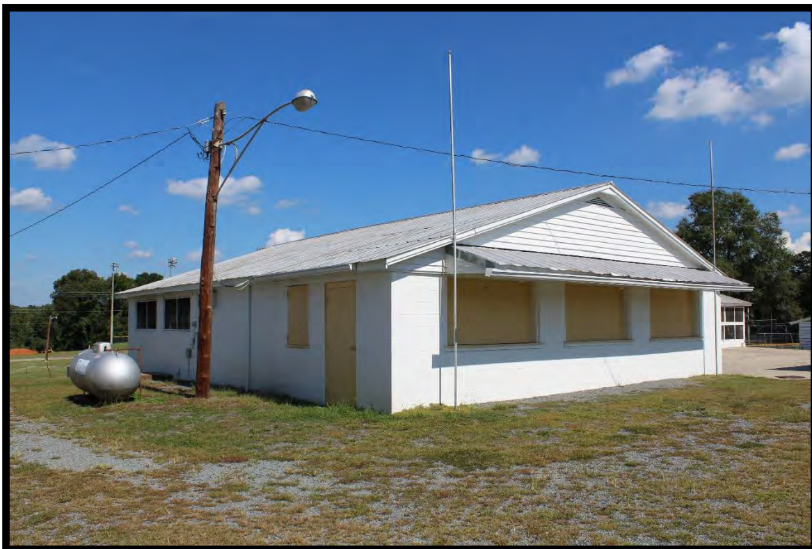
Figure 12: Sandwich Stand, Mallard Creek School, Looking Northeast.
