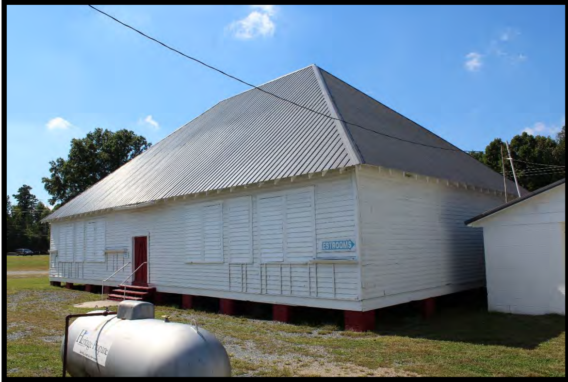
Figure 8: Mallard Creek School, Looking Southeast.
