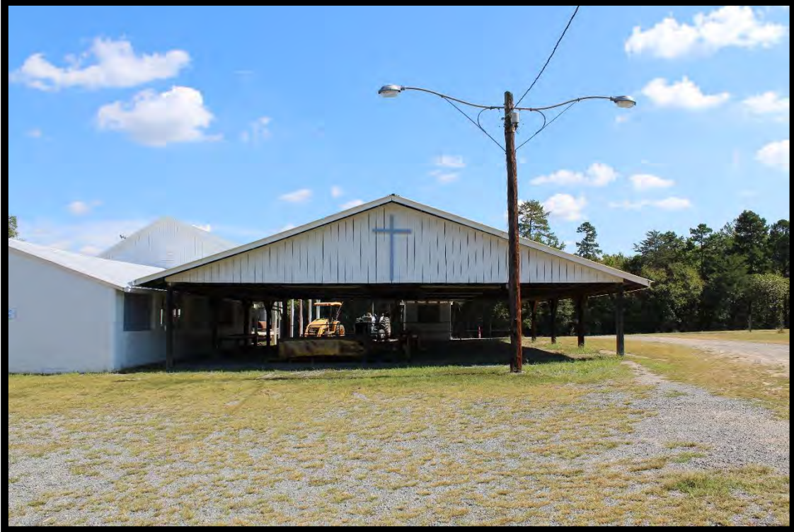
Figure 18: Picnic Shelter, Mallard Creek School, Looking East.
