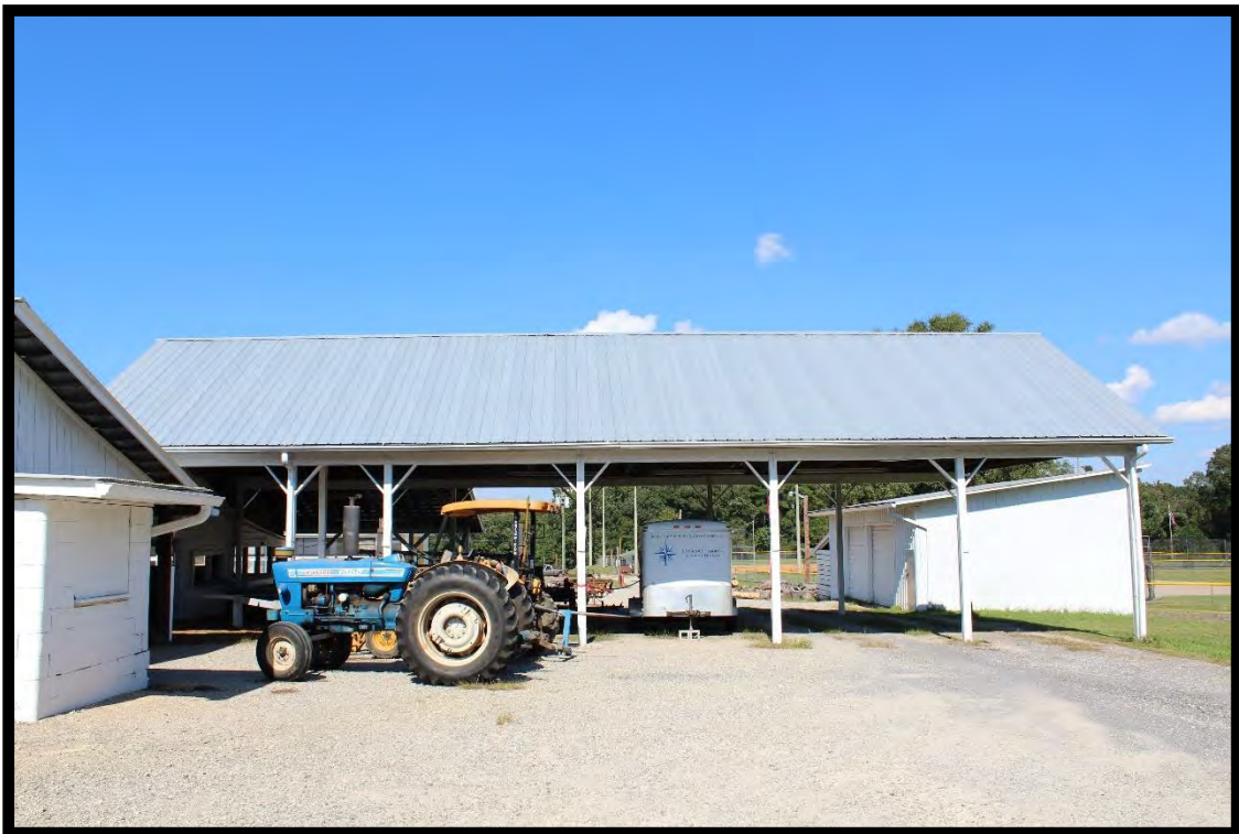
Figure 21: Drive Through, Mallard Creek School, Looking North.
