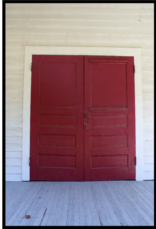
Figure 5: Entry Door, Mallard Creek School, Looking East.
