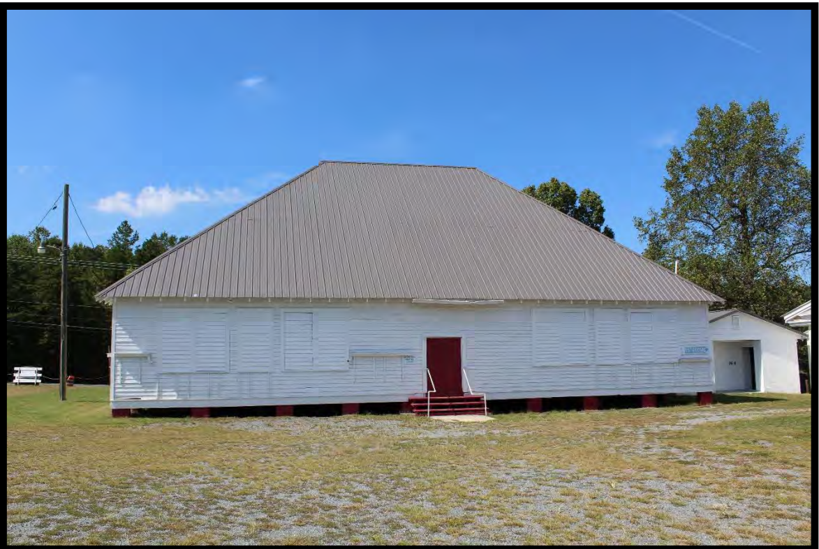
Figure 7: Mallard Creek School, Looking West.
