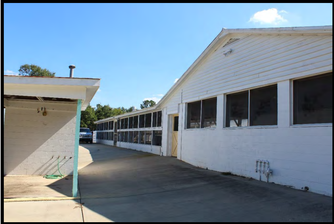
Figure 13: Sandwich Stand and Barbecue Building, Mallard Creek School, Looking Southeast.
